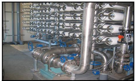
Figure 5: Oxnard Desalter's Two Stage 46x23 RO with ERD Turbo Booster
