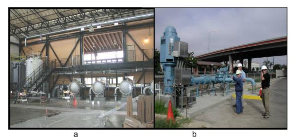
Figure 1: Oxnard's High-Pressure Cartridge Filtration System and Well Pumps
